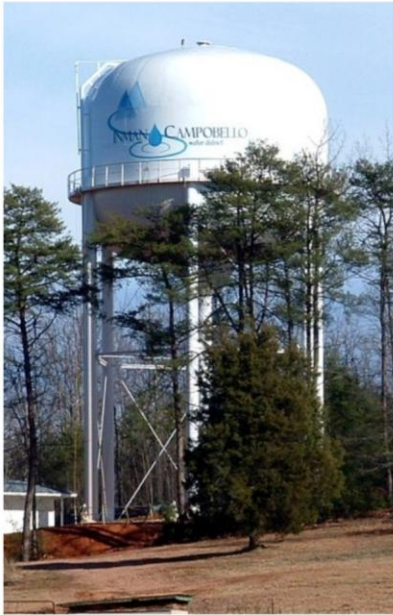
New ICWD water tank—Firetower Rd.
